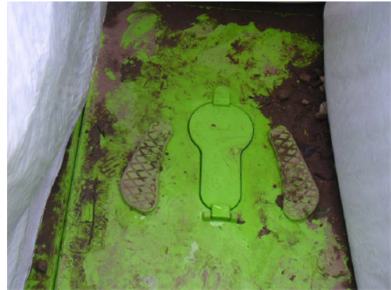
Platform in latrine tent
